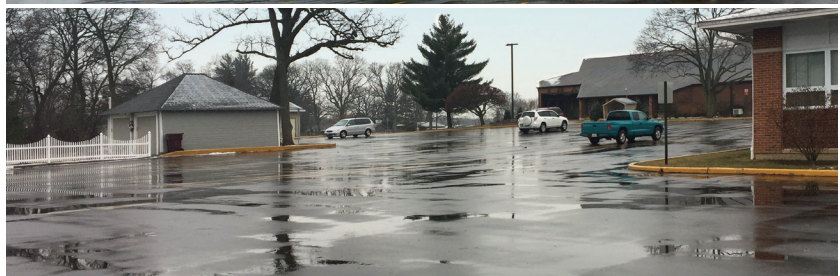
St. Joseph parish used campaign funds to renovate the church's parking lot and repair the roof.
